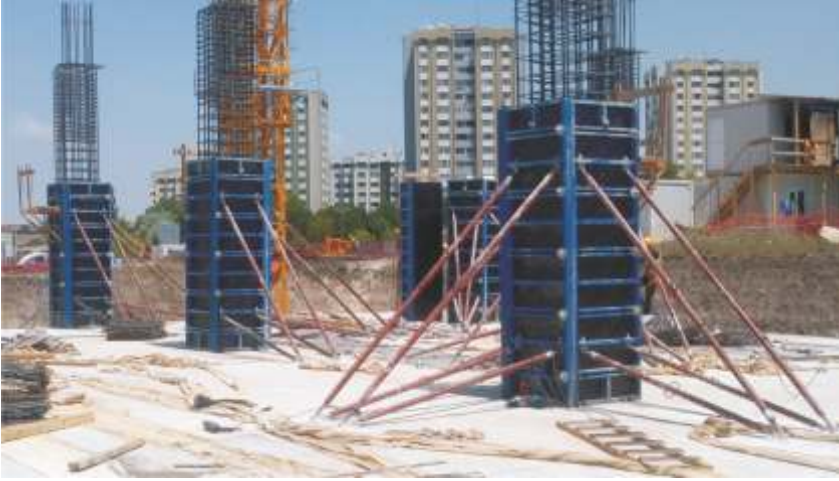
Combination of MO-KAI panels side by side which are used on current column, it can be launch reliance curtain or building curtain
